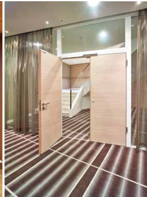
Double-leaf door to the stairway.
