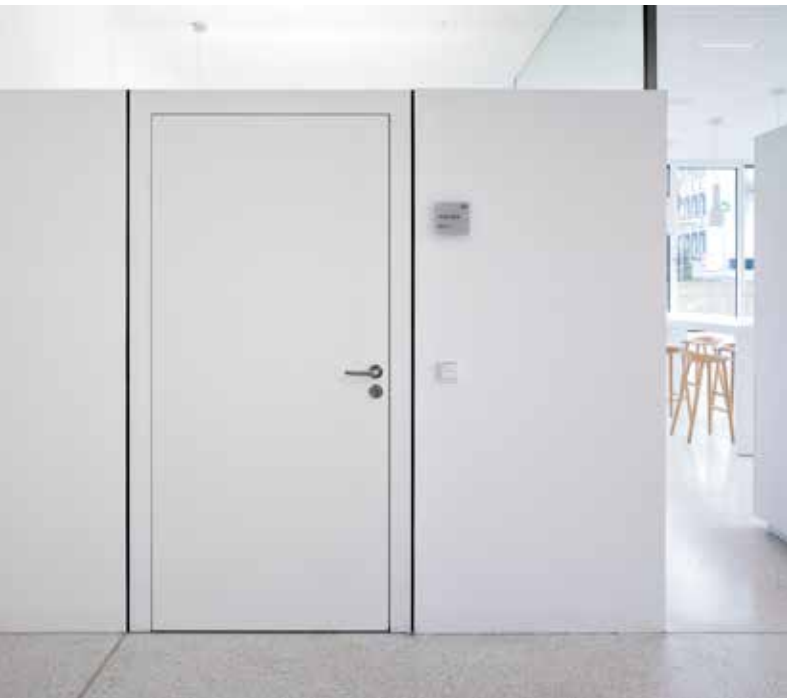
Schörghuber office doors are flush-fitting with the wall. The subtle black gaps highlight the doors – including those to secondary rooms.
