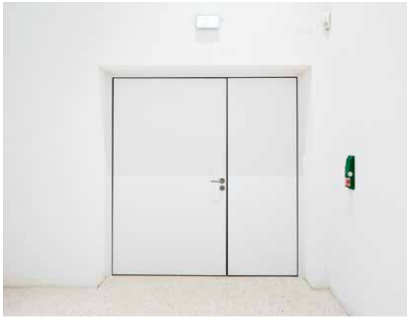
If necessary, the fixed leaf can be opened to extend the passage.
