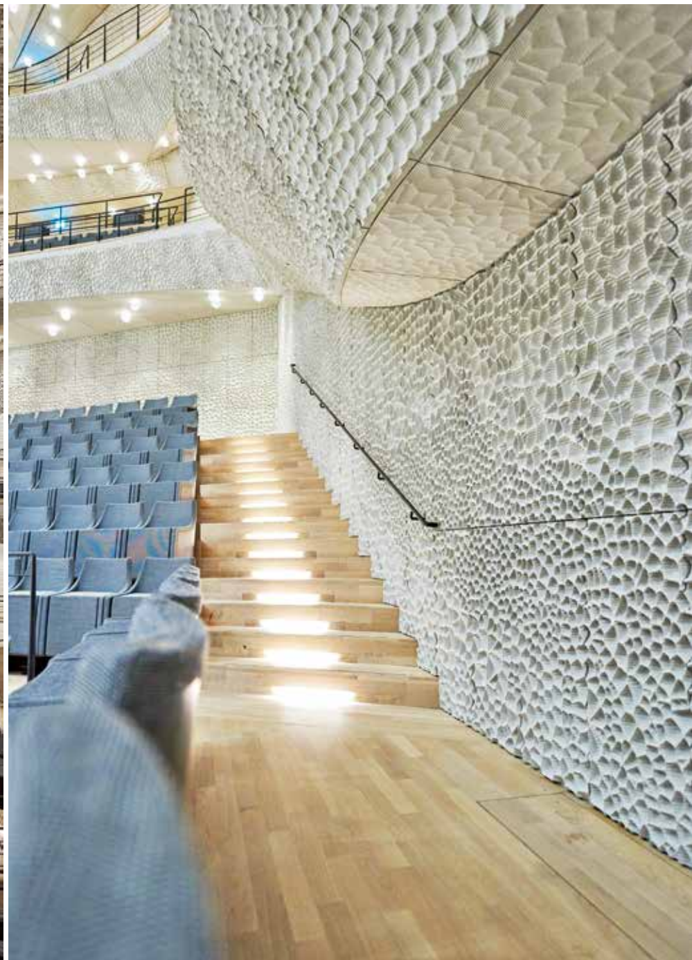
Acoustically effective: the "white shell" of the Large Hall made of specially milled gypsum boards.
