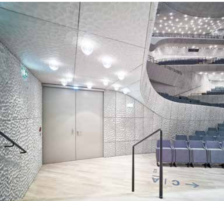
Double-leaf fire-rated and smoke-tight doors in the Large Hall.
