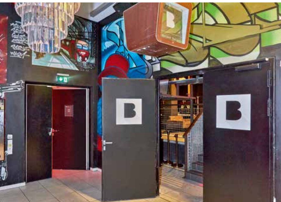
In the background, another T30 fire-rated and smoke-tight door leads to the stairway.
