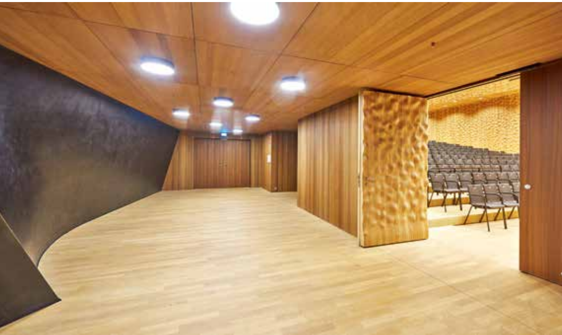
The Small Hall as well as the Schörghuber doors are lined with specially milled oak boards.
